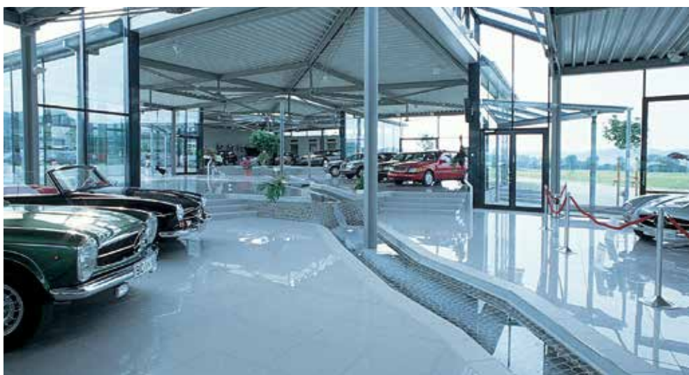
Roth radiant heating and cooling system, Auto Velte KG car dealership, Biedenkopf, Germany
